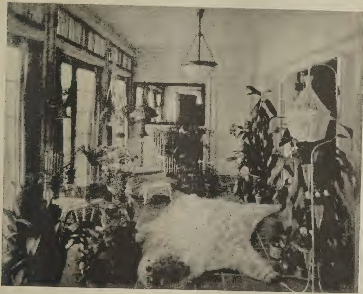
NOTE THE VENTILATORS ON THE LEFT SIDE. SEE THE DETACHABLE SAUCERS UNDER THE PLANT POTS. THE TILE FLOOR IS GOOD, BUT THE LARGE RUG IS SUPERFLUOUS. THERE IS PROBABLY A DRAIN AT THE LEFT, AS THE FLOOR SLOPES TOWARD THAT SIDE. A DOOR AT THE RIGHT FACILITATES REGULATION OF TEMPERATURE. THE HANGING BASKETS ARE FIRMLY SUSPENDED. THE LARGE RADIATOR AT THE REAR SHOULD GIVE PLACE TO PIPES RUNNING HORIZONTALLY AROUND THE ROOM. THE PLANT STAND IN FRONT OF IT IS FULLY DESCRIBED ON PAGE 43
